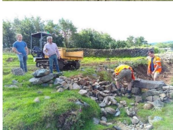
Improvements were also made around a yard area lower down, which was affected by the flood water. Water was diverted away from cattle feeding and loafing areas and bunded areas created to intercept the water. Trees suited to the wet conditions were planted to help with water infiltration, screening and biodiversity.
