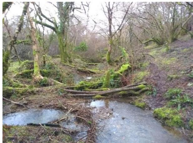
**Live willow faggot dams** are naturally leaky and provide a great barrier for slowing water, trapping silt and debris and with the advantage that the willow faggot and stakes will grow (below right). This will further stabilise the structure, the roots will help with water infiltration and absorption and there are habitat and livestock health benefits from willow too.
