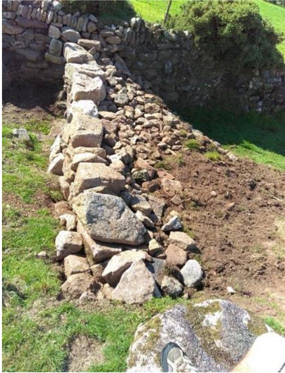
**Stone dams** vary greatly according to their location and function and are most suited to ditches or gullies with surface water flows where the passage of fish will not be impeded. The stone structure is built to be deliberately leaky to allow the passage of normal flows.
