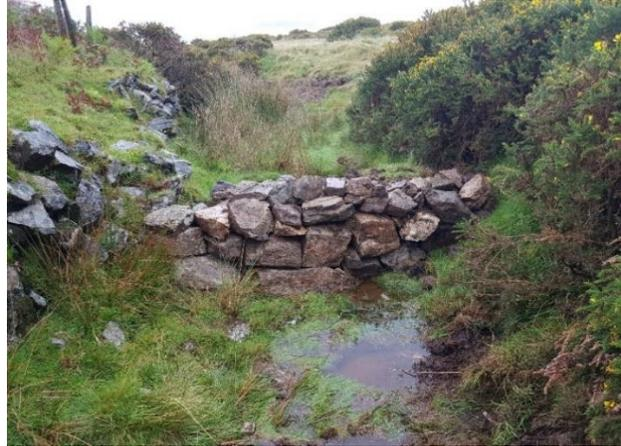
Water permeates slowly through the smaller stone on the downstream side of the structure, preventing erosion from any great force of water. These stone dams stood the test of storm Dennis, overtopping but without the loss of any stone.
