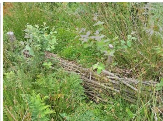
Willow faggots can be adapted for use in a variety of situations. In this very steep, incised gully faggots were used both to create frequent leaky barriers across the width of the gully and are also pegged down lengthways into deeply eroded channels and erosion holes to prevent further damage.
