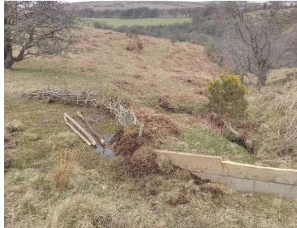
On the right timber boards are used to slow and channel flows in combination with willow faggots used to hold water and to enhance wetland habitat. Timber is a useful material to use in situations where the gully bed is too dry for live willow faggots or where a more robust structure is needed. These dams do not always initially blend into the landscape as well as other types but will weather in time.
