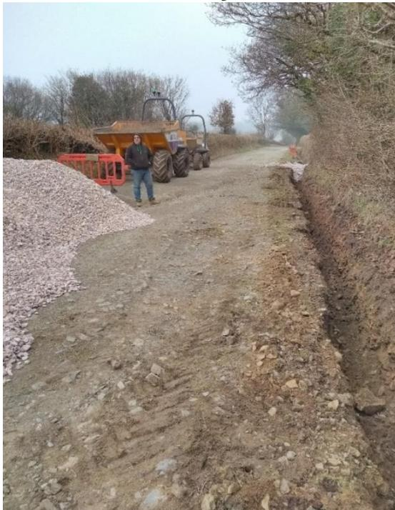
Houses in Scorrilton have been flooded very recently as a result of flood water running down the driftway into the village. In a joint project between the Ranger Service and the Headwaters Project drainage improvements have been carried out, to include new French drains, renewed cross drains and a series of trial infiltration pits to soak away the water.
