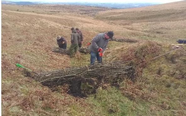
Leaky dams made from both live willow faggots and timber boards were installed into a network of old tin mining gullies, many of which channel significant flows during heavy rainfall.
